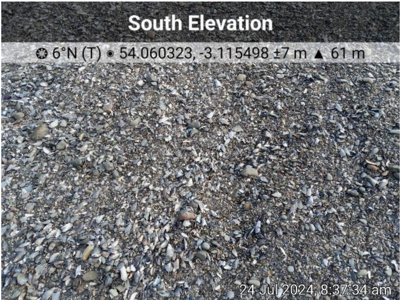
Figure 22. Raised bank consisting mainly of shell debris and stone 24-07-24
