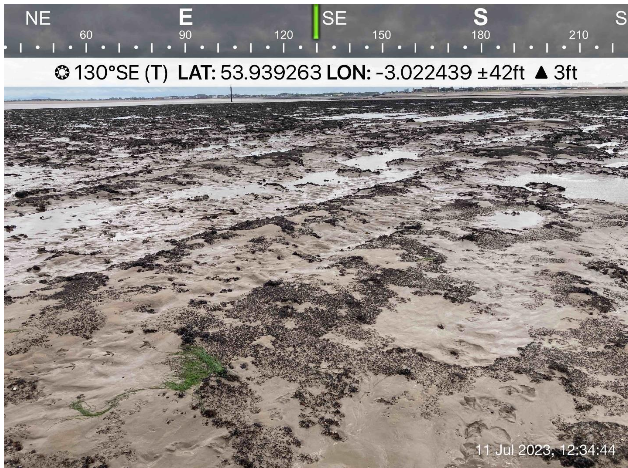
Figure 6: Perch Scar evidence of scour.
