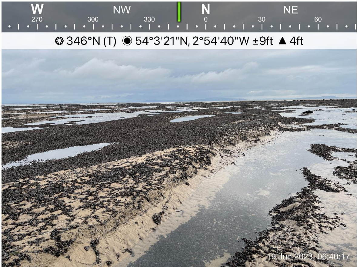
Figure 4. Evidence of scour and loose seed mussel Heysham Flat 19-06-23.
