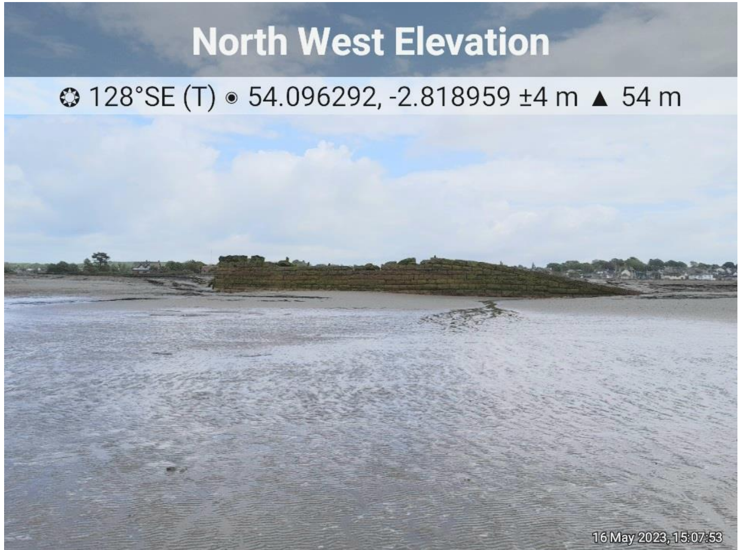
Fig 1 – Previously buried structure, now 2.5m above surface
